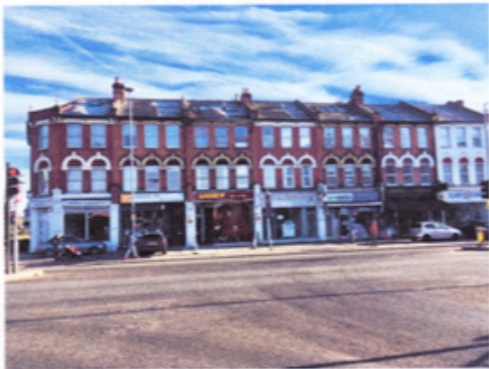
74-84 Richmond Road - Locally Listed Buildings
