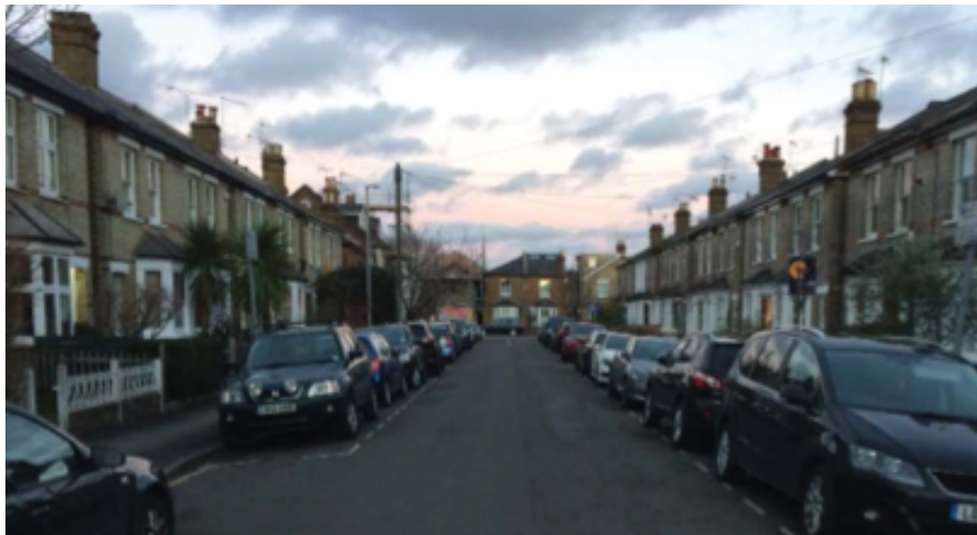
Osborne Road: Victorian houses with well maintained typical architectural features
