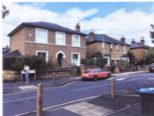
Gibbon Road - south
